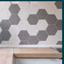
DADO CERAMIC TILES 600 MM ABOVE THE COUNTER
